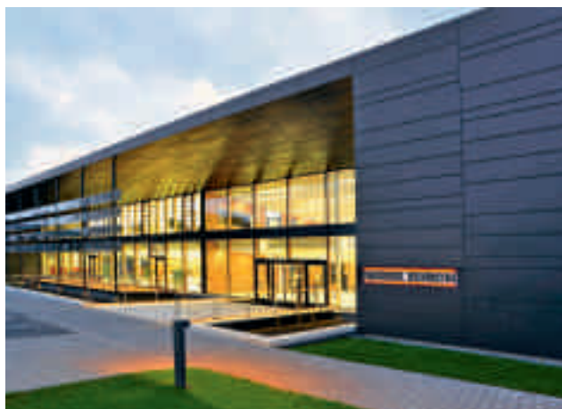
6 | Energy Campus in Holzminden
